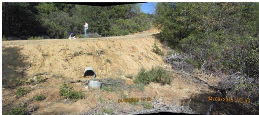
Image 16 – Crossing C4 outlet – note evidence of runoff and erosion over the side of the road at this location. (Photo 9006)
