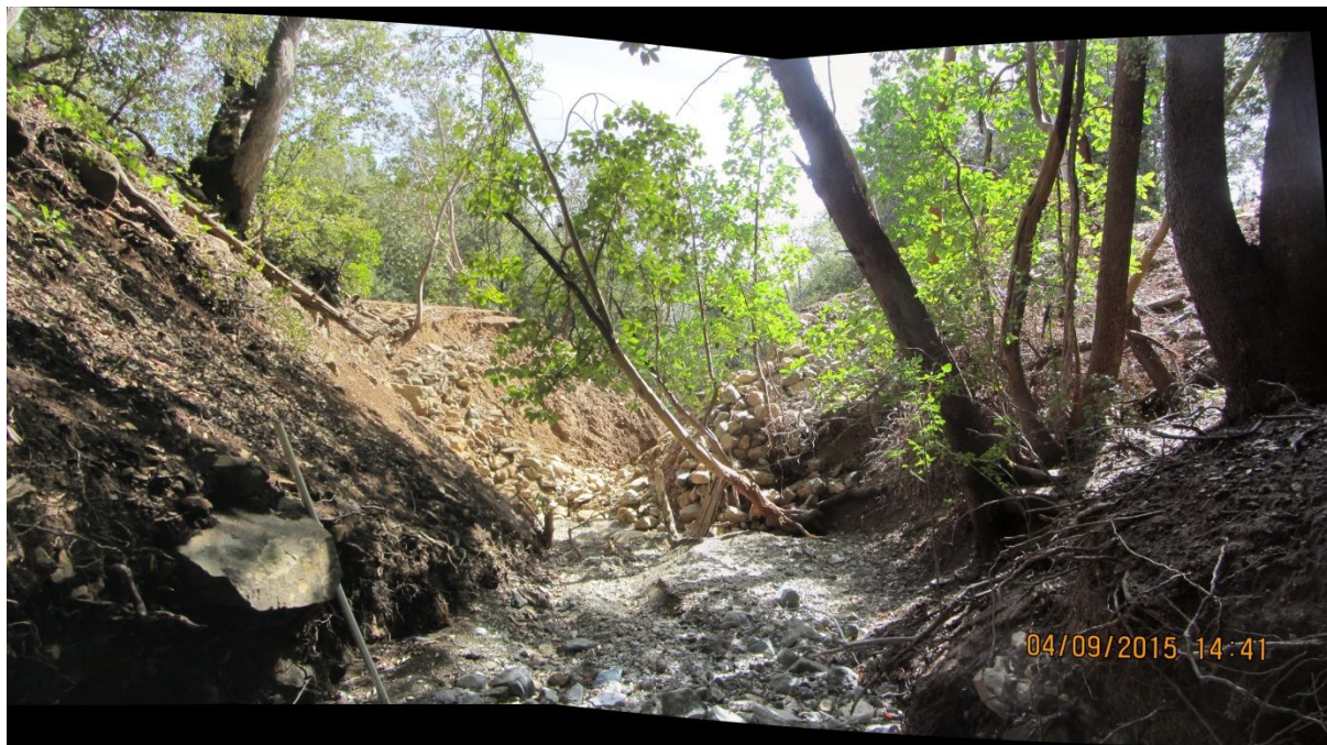
Image 9 shows Crossing 3 and the eroded fills looking downstream. (Photos 8971, 8972, 8973, 8974, 8975, 8976 composite)
