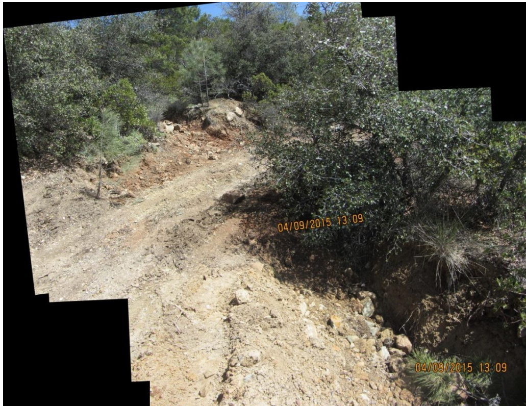
Image 1 shows crossing 1 (C1). Note the earthen fill in the stream channel and perched along the road at the outlet. (Stitch of photos 8925, 8926, 8927, and 8928)
