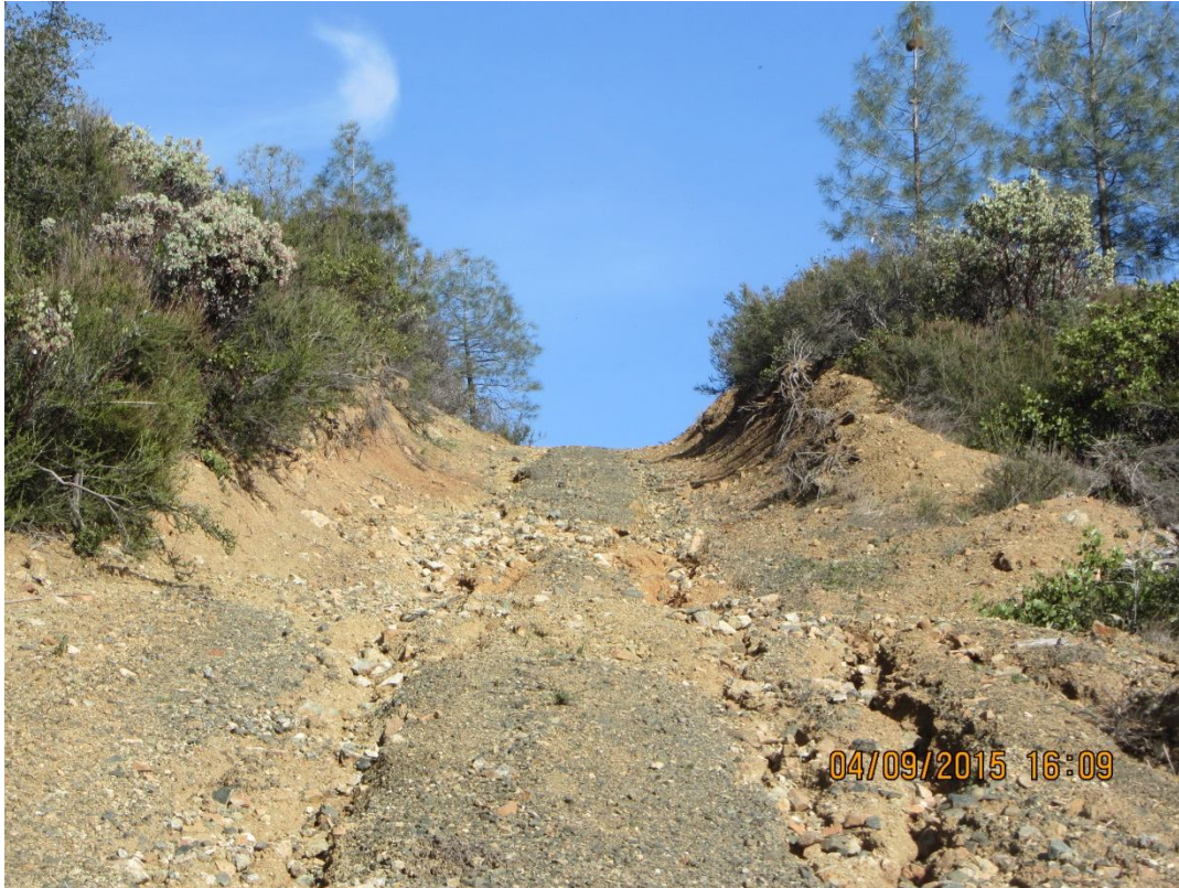
Image 18 – Road segment 1 – a closer view of the through cut at the top of the ridge that starts the concentration of flows and encourages road surface erosion. (Photo 9044)
