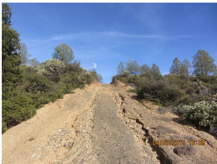
Image 17 – Road segment 1 – shows erosion on the road surface looking east toward the through cut. (Photo 9043)
