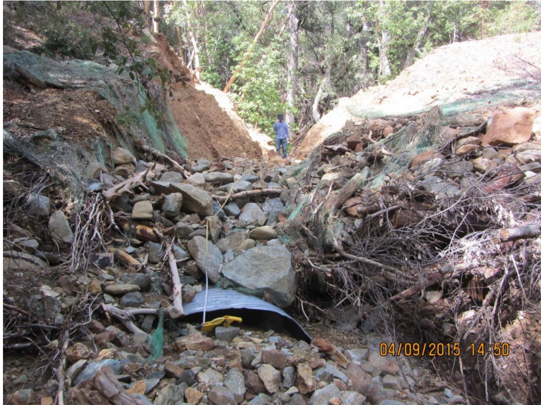
Image 10 shows Crossing 3 looking upstream; note the erosion control fabric displaced on the side slopes of the crossing from fill failures, and the culvert buried in the foreground. (Photo 8980)
