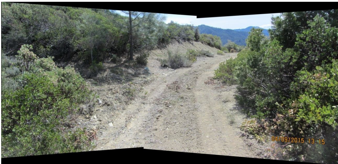
Image 3 - the road surface at point C2. Note that this crossing shows little effect from the winter rains. This stream is near the ridge top and likely is influenced by large storms but not minor rain events. (Stitch of photos 8936, 8937)
