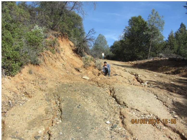
Image 15 = Road segment 1 – shows the erosion on road surface. (Photo 9018)
