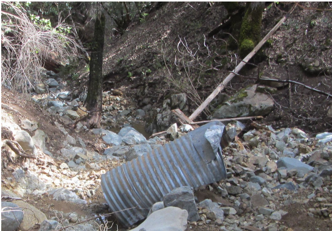
Image 13 shows a section of the 54" culvert torn out and displaced downstream from Crossing 3. Note that there does not appear to be any evidence to indicate the culvert was installed with a flange of angle iron as specified in the 1600 application, and as would at minimum be required to maintain the culvert in the stream if it were sized adequately. (Photo 8988 cropped)
