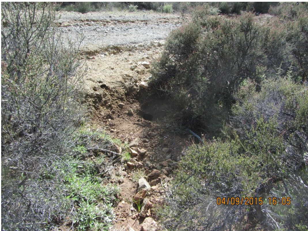
Image 19 – Crossing C5 inlet. C5 is a 6-7 inch flex pipe, undersized for this crossing. The inspection team excavated the inlet in order to photograph the pipe. (Photo 9040)
